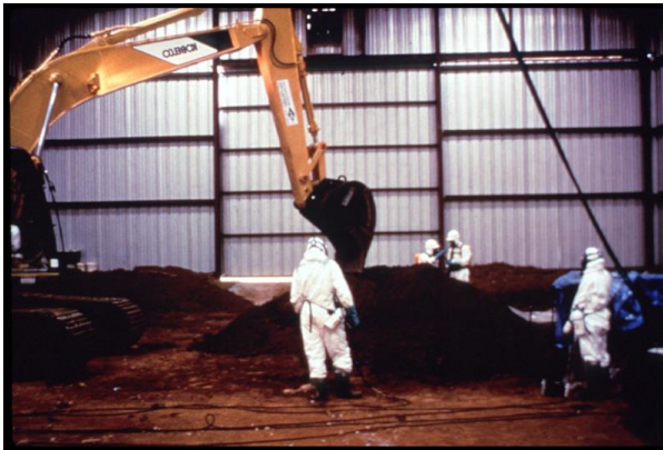
Contaminated soil excavation
